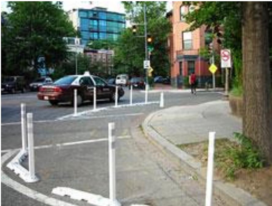
*Figure 1. Panel and Bollard bumpout, example*
